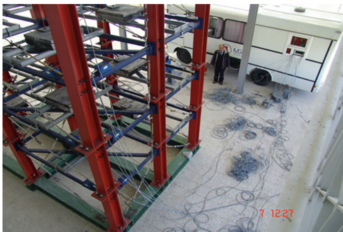
Fig. 10.1 Mobile structural monitoring system and steel frame benchmark structure
